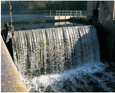
Fig. 1. A mobile spillway gate on the Sambre river
